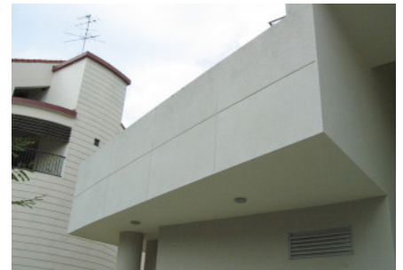
Building services enclosure with exterior paint finish
