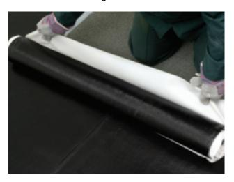
Figure 2 Application of Self-Adhesive Membranes
