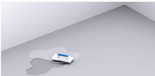
**1.** Clean and prepare the surface with self-levelling mortar ARGONIV® 020 or ARGONIV® 120, eliminating unevenness.
