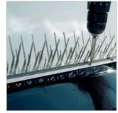
5. Install on window ledges, conservatories etc. It is recommended that sealant is used around penetrations to make watertight.
