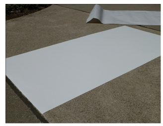
F. Apply all panels, aligning to previous panels and axis lines. Weed out design to expose concrete for your application.
