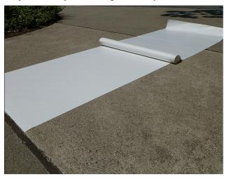
E. Measure panel placement to main axis & 90 degree lines. Smooth down panel and assure even adhesion to surface.
