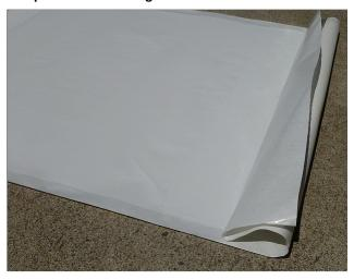
B. Align panel to straight edge and apply to surface.
