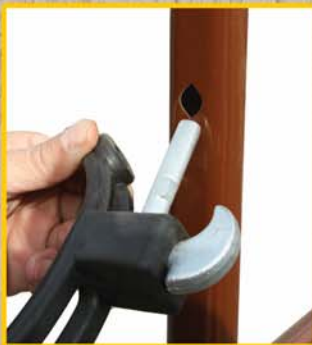
1. Insert pin into panel with hook on the outside (non-animal side) of the corral.
