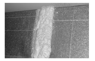
FIGURE 1—DUCT JOINT SEALING
