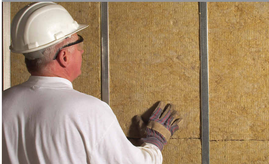
Thermafiber SAFBs are installed into an interior steel stud wall cavity.
