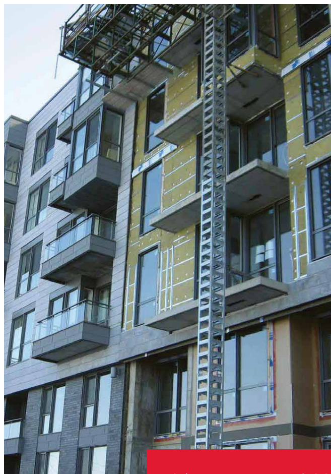
Soleno Project, Montreal, QC ROCKWOOL CAVITYROCK®
