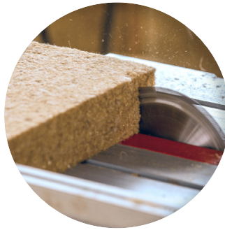
Cutting the Insulation
