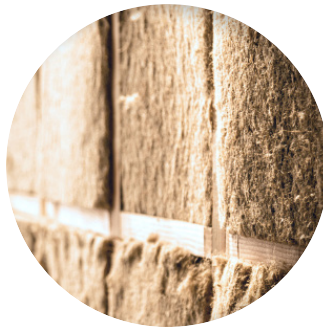
Installing Between Studs
