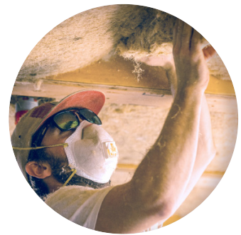
Possible Second Layer (Cross-Jointed)
