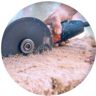
Insulation Cutting
