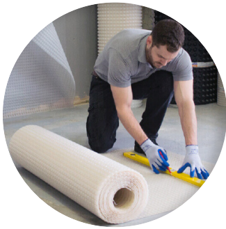
Prior to Installation
