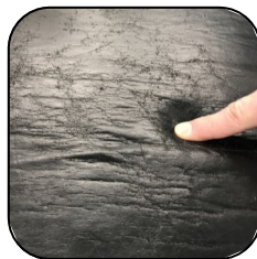
Extensive Cracking
