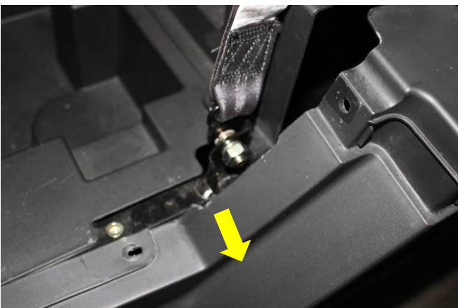
Main panel pulled outward
