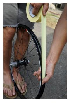
Ensure that you have a firm grip on the tape's end as you apply ample tension when setting WTB TCS rim tape into the WTB TCS rim trough.
