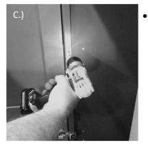
mark the first two vertical holes in the slide on to the frame. Then temporarily remove the slide again and set aside.
