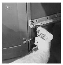
Replace the slide into the back support, place the provided spacer between the frame and slide, and screw into place. Repeat steps for both sides. Then continue to Step 4.
