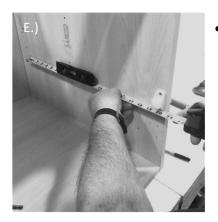
Using a tape measure and level, measure 20 ½" from the edge of the cabinet and make a crosshair mark at that point and at the height previously chosen. i.e. 6" in the pic.
