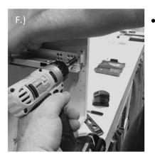
Install the slides onto the 1" spacers, repeat all Option B steps A - F for the other side, then continue to Step 4 below.
