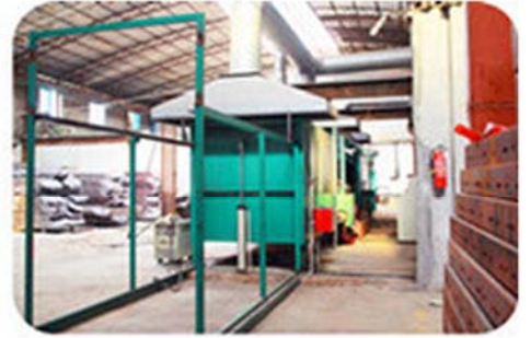
PVC Coating Workshop
