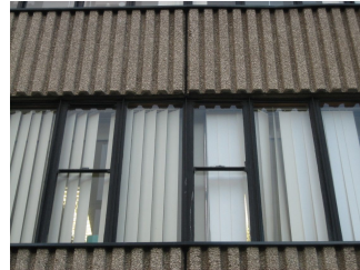
1970s concrete frame office with poor performance
