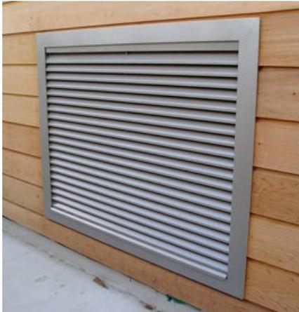
Figure 4 – Ventilation louvre (Passivent©)
