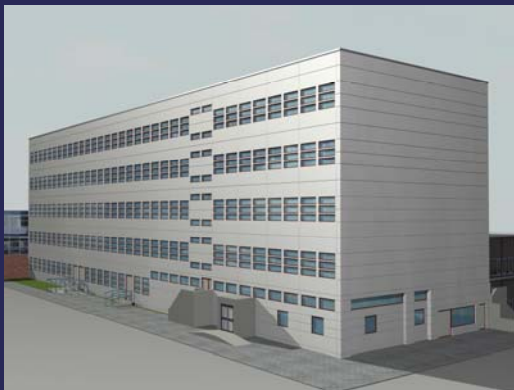
Visualisation of OBU Building After Over-Cladding
