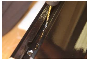
Figure 32: Pilot the holes with a small drill bit
