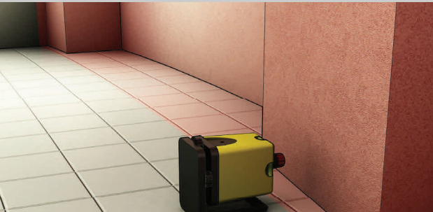
Determine greatest projection (Bump out in wall) to determine face of panel floor layout lines.
