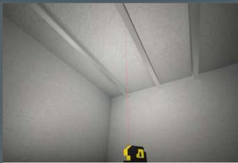
Use a laser level to transfer the cable connection points to the ceiling structure.
