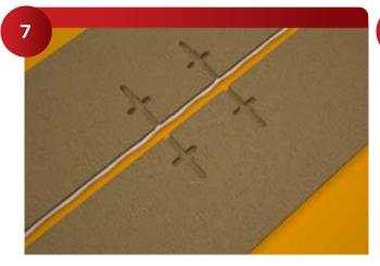
To join the countertops, apply a generous amount of silicone or other waterproof glue to ensure the seam is waterproof and never moves.
