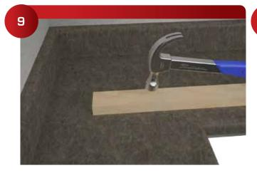
Use a wood block to hammer the countertop flush prior to the final tightening.
