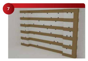
Using a 3rd ¾" thick block, work down the line, one stud at a time to level, shim, glue and screw the furring into permanently into place.
