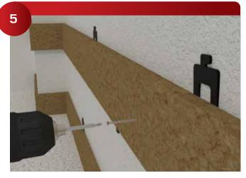
Use a level, shims and glue to screw and lock the far left and right sides of the furring into place. This provides level work surfaces to straighten the middle of the furring.
