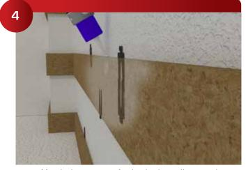
After laying out your furring horizontally, start the installation of the furring systems by nailing the furring straight into position, without panel adhesive. This allows the furring to be adjusted in and out.
