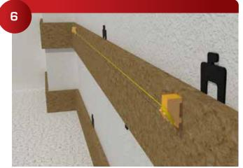
Place a <sup>3</sup>/<sub>4</sub>" thick blocks on the far left and right sides of the furring that are fixed and leveled. Pull a tight string line between the blocks.
