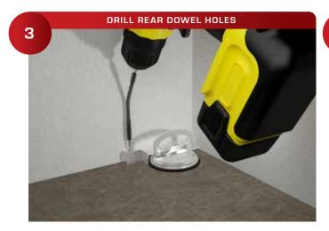
Use the Backsplash Drill Jig to drill 5/16" dowel holes in the low and recessed areas of the wall and countertop, about 36" OC should work.
