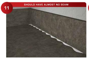
At this point your Backslash should have almost no seam and be securely locked into place with gap between the backsplash and the countertop 100% filled.
