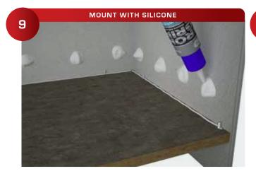
Place a thick bead of silicone on the wall above. The goal is not to let the silicone ooze over on the wall, most wall paint will not stick to silicone adhesive.
