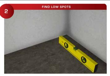
After the countertop is securely installed, find low points and the recessed areas of the drywall of the countertop with a level or straight edge.
