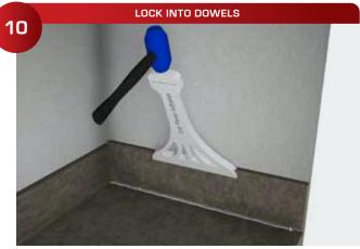
Force the backsplash down onto the dowels and into the bed of silicone. Lock into place with a dead blow hammer or clean block. (**Useful Assesories:** The 920 Panel Adjuster works well here.)
