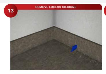
Using a soft plastic chalk scraper, scrape off all the excess silicone. This should leave a fine, clear, water resistance line of caulk.
