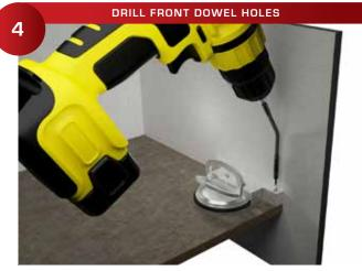
Drill dowel holes about 4" from the front end of the backsplash.
