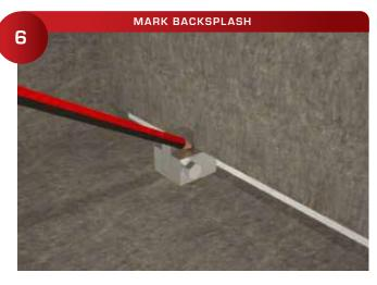
Dry fit the backsplash into position and make the pencil marks on both sides of the dowel to the backsplash.
