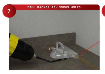
Using the pencil marks as your guide for the Backsplash Drill Jig, drill the holes for the Dowels.
