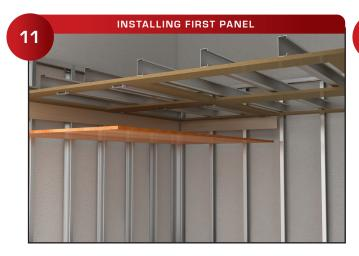
Pretest the fit of the ceiling panel carefully and make sure each clip is properly placed before installing the Locking Arms.
