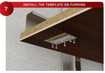
Use a small nail gun or screws to install the Plywood Template securely and accurately onto the furring. Push the upper clip to the back of the guide pocket and screw the clips into place.
