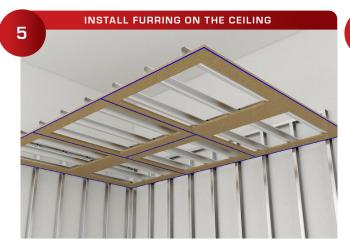
Install the furring securely onto the structure above, the furring does not have to be precisely installed. Transfer your panel layout from the floor to the furring.
