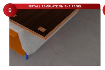
Use a small nail gun or screws to install the Plywood Template securely and accurately onto the panel.
