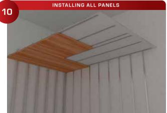
The ceiling clip allows for about ¼" of movement. (**Tip:** The ceiling panel can be glued with a small spot of silicone to hold reveal tolerance.)
