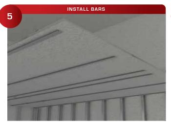
Install the 511 Ceiling Clip Bars, shim if needed to a plate plane. Use 2 screws at bar joints. (Recommendation: Hilti Self Drilling, Self-Tapping Screws at every stud.)
