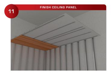
The panels are now safely in place and still permanently removeable.
