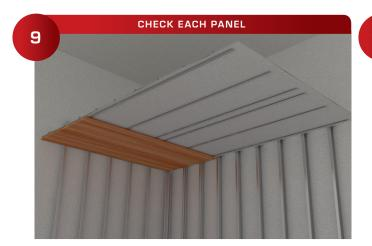
Install the ceiling panel carefully and make sure each clip has dropped into place.
