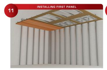
Install the ceiling panel carefully and make sure each clip has dropped into place.
