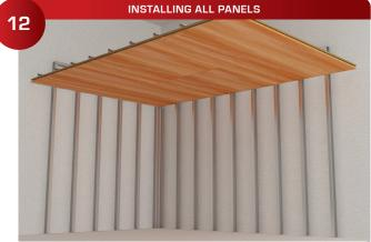
Ceiling panels can be glued with a small spot of silicone to hold reveal tolerances. The panels are now safely in place and still permanently removeable.
