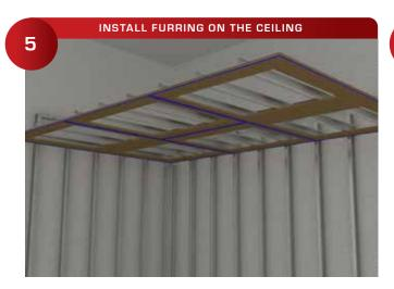
Securely install 3/4" plywood furring with a string line. level & flat.
