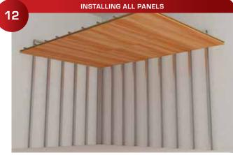
Ceiling panels can be glued with a small spot of silicone to hold reveal tolerances. The panels are now safely in place and still permanently removeable.
