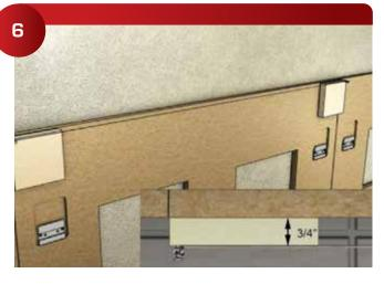
Use a string line to straighten the pre-cut furring. (Tip: If you have per-glued the furring panels, you need to work quickly.)
