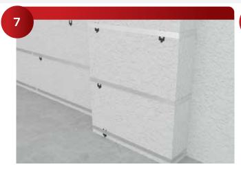
Starting in the corners shim the bars out to the greatest projection per wall, then use a string line to straighten each bar between the corners. The finished bars should be level and straight.
