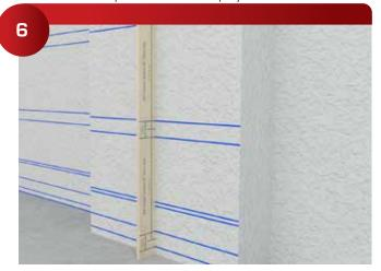
Layout a story pole that includes the benchmark, top and bottom of the Bars and Clips, they are 3" apart. The bars should be about 24" apart. Proceed around the space marking at the bottom of the clips at every stud.
