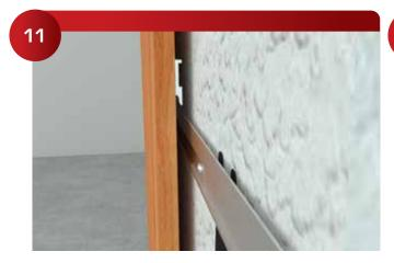
Lift the panel into place about 1/2" above marks, push in and down firmly to lock the panels into their final position.
