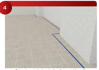
Determine greatest projection (bump out in wall). This will determine the face of the panels. If there is a large bump, discuss the layout options with the GC. There are generally two options, shim out your 430 S Clip Bars or have the projection corrected.
