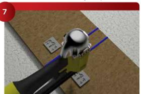
Screw or Staple the 400 NZ Clips at all corners and 24" on center or as needed.
