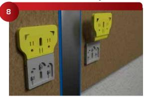
Place 410 NZ Alignment Clips on each individual panel's set of clips (**Tip:** The 410 NZ Alignment Clips are reusable.).
