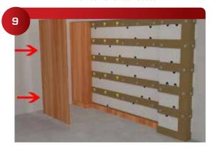
Place reveal spacers between panels to locate the exact panel positions. Carefully push the panel into the 410 NZ Alignment Clips to mark the panel clip position.
