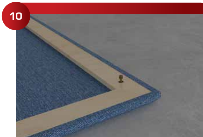
Drill a 1/2 hole in the positions indicated by the 211 Alignment Pins and press in the 349 Upholstery Mounts.
