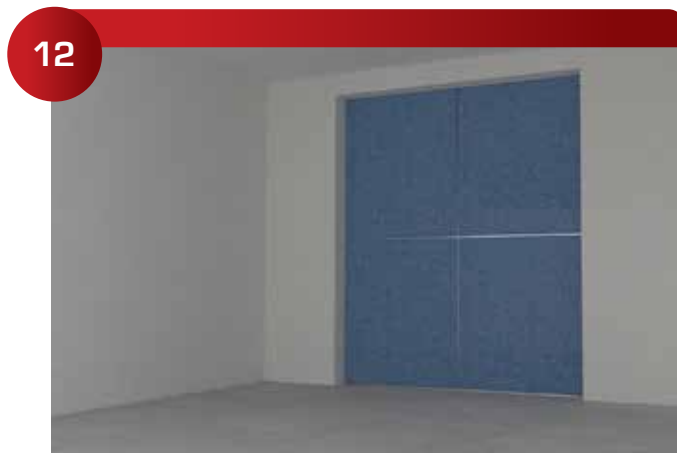
Completed Panel System.
