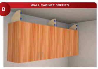
Install wall gussets above the wall cabinets with the 325 Zero Side Mounts pre-installed. The gussets can be installed by simply sitting them in beads of panel adhesive and allowed to dry overnight.
