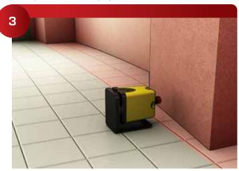
Determine greatest projection (bump out in wall) to determine face of panel horizontal layout. Determine panel widths based on horizontal lines and field alignment requirements
