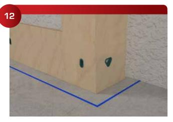
Adjust and set plumb all corners and outside edges of the prefabricated panel furring. The installation and fit of the prefabricated panel furring will verify the fit of the panels.
