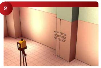
Carefully review the shop drawing to understand field alignment requirements. Find high point of the floor and set horizontal bench mark at any workable point.
