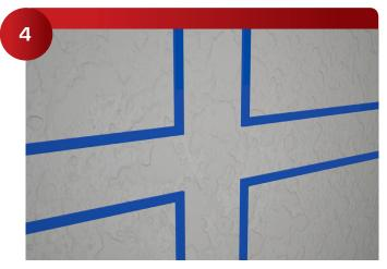
It is helpful to offset the panel location blue chalk lines by 1/2" wider than the reveals. This provides the layout for the installation of reveal laminate strips later in the process.
