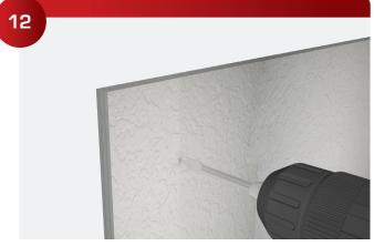
Using ½" sharp flat bit slowly drill the drywall holes in the appropriate locations.
