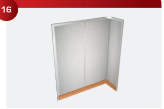
Install reveal strips between the chalk lines with contact cement. The joints can be cut with laminate shears.
