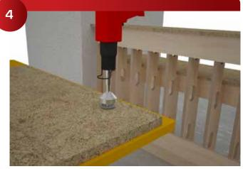
The 225 Galaxy can be plant installed flush with the furring. A plant prepared CNC cut die wall parts, including the 5mm holes for the mounting screw makes the field installation very quick.
