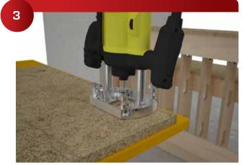
The 225 Galaxy can be field installed using a 911 Carbide Tipped Drill 1-1/4", Forstner Drill. However, most solid surface manufactures prefer the holes be cut with a router to avoid heat buildup.
