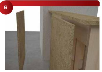
Carefully place the panel in the correct position and bump the panel in each corner to mark the location of each mounting screw.
