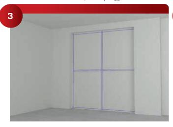
Layout the perimeter of the panels on the walls with a blue chalk line. Confirm that the panel layout is workable with field alignment, electrical and any other requirements.
