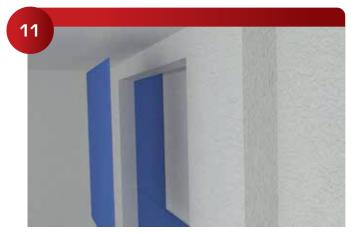
To install the panels they must be carefully realigned with the mounting screws. Then push them straight into place firmly, you should hear them click and lock in position. (TIP: Use reveal spacers to quickly locate the position of the panel.)
