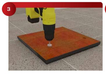
The 226 Galaxy can be field installed using a 911 Carbide Tipped Drill 1-1/4", Forstner Drill
