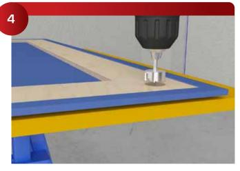
225 Galaxy should be drilled about 2" off the panel corners to firmly hold the panels. Drill the holes with a 911 Carbide Tipped Drill 1-1/4", Forstner Drill, 3/8" deep.
