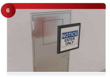
Carefully place the sign in the correct position and bump the sign in each corner to mark the location of each mounting screw.
