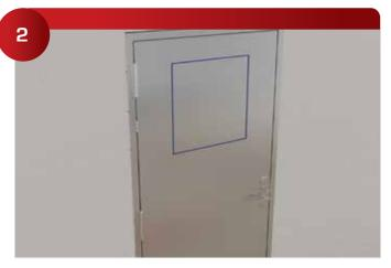
Determine the location of the sign and lightly mark the location, use tape on the door if it's too hard to mark.
