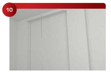
The reveals can be quickly painted, or you can use 1/32" plastic laminate with contact cement.
