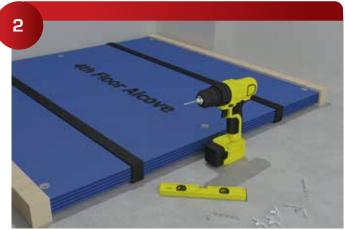
When shipped in a pre-assembled flat packed kit, the tools required for customer installation are minimal. Tools required for "Customer DIY Installation": 229 Galaxy Alignment Pins, 236 Combination Screws, 919 Carbide Tipped Drill 5/16", 911 Carbide Tipped Drill 1-1/4", 952 Pop Toggle.
