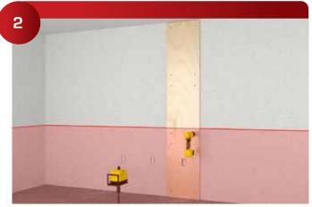
Cut a ¾" wood template, sized to the centerline of the reveals. 917 Drill Collars can be used to improve durability and precision. The 224 Galaxy should be drilled about 2" off the panel corners and every 24" to firmly hold the panels.
