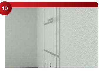
Install reveal strips with contact cement or paint over the chalk lines. The joints can be cut with laminate shears.
