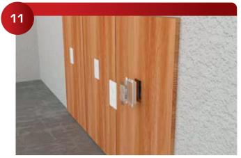
To install the panels they must be carefully realigned with the mounting screws. Next push them straight into place firmly, you should hear them lock in position. (TIP: Use spacer strips to quickly locate the position of the panel).
