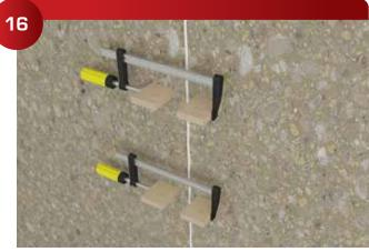
Use bar clamps to force the panels together, floating on the silicone. Push the panel into place with a dead blow hammer until all areas of the panel are set in the silicone. To alignment the panels, (vacuum cup alignment tools are available for this step). The Galaxy 226 will flex enough to work the seam.
