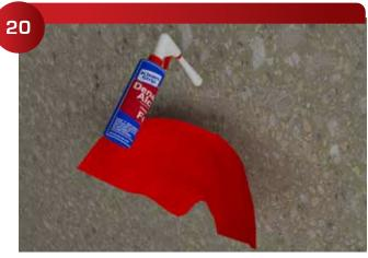
Clean the surface and caulk perimeter of the wall with paintable clear caulk.
