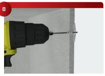
Install the 952 Pop Toggle into the sheetrock, it should fit firmly. Push the setting stick into the 952 Pop Toggle to get the arms to pop out. Using a drill set on low torque, gently snug the 236 Combination Screws into the 952 Pop Toggles. The gap between the sheetrock and the solid surface panel can be adjusted with the screws or washer. Most solid surface manufacturers recommend 1/8" gap.
