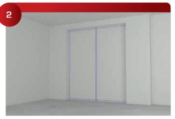
Layout the perimeter of the panels on the walls with a blue chalk line. Confirm that the panel layout is workable with field alignment, electrical and any other requirements. Tip, the sheetrock finish should be Level 2 only, taped, one coat, no corner bead, no skim coat.
