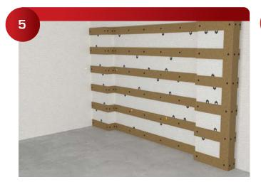
Using string lines or a laser, shim, glue, and screw all horizontal furring into place.
