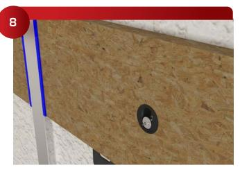
Place 211 Alignment Pins in each Lock needed to mark one full panel.
