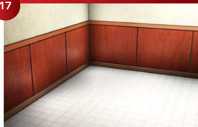
Finished paneled wall.
