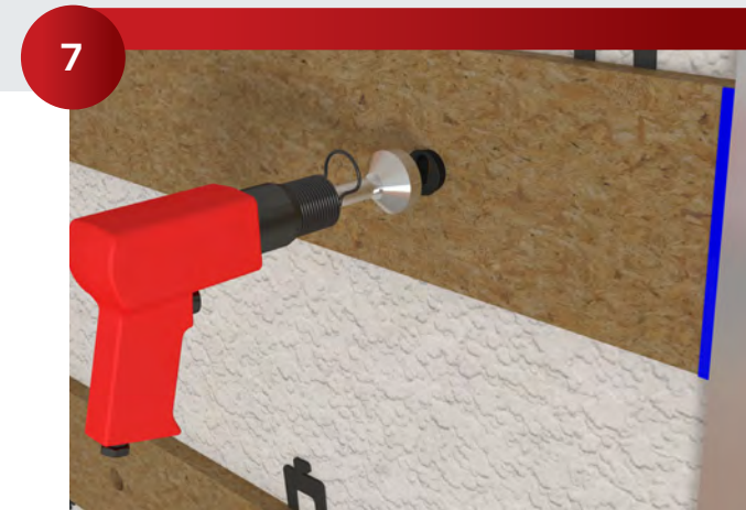
Insert the 210 Lock at 24" on center or as needed. The Locks can be drilled to 1" with a 910 Carbide Tipped 1" Forstner Drill, Center Point Drill
