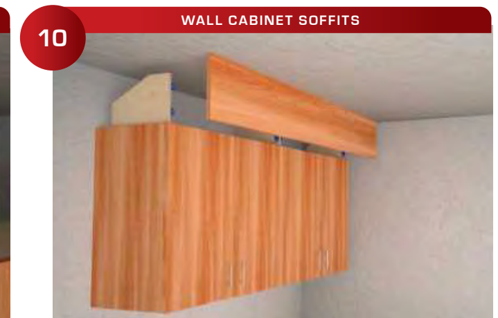
Push the soffit firmly against the 330 Zero Alignment Pins to mark the 334 Mounting Screw locations.
