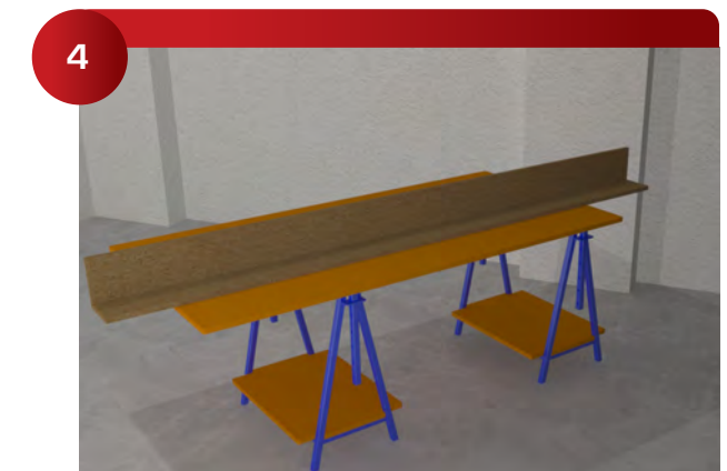
Preassemble the vertical furring corners (if any) and install them to use as a guide for the horizontal furring.
