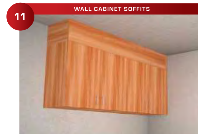
The completed soffits above the cabinets can be removed for later access.
