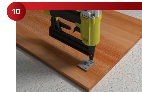
10 Screw or staple the 400 NZ Clips in the position indicated by the Alignment Clips. ( Tip: You have the option of using only the center slotted screw if you need the clips to be adjustable.)
