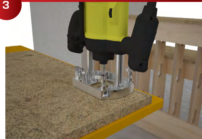
The 225 Galaxy can be field installed using a 911 Carbide Tipped Drill 1-1/4", Forstner Drill. However, most solid surface manufactures prefer the holes be cut with a router to avoid heat buildup.
