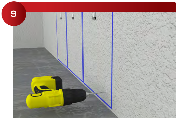
Using a drill set on low torque, gently snug the 236 Combination Screw into the 952 Pop Toggle. (TIP: Do not over tighten the screw, it can compress into the sheetrock.)
