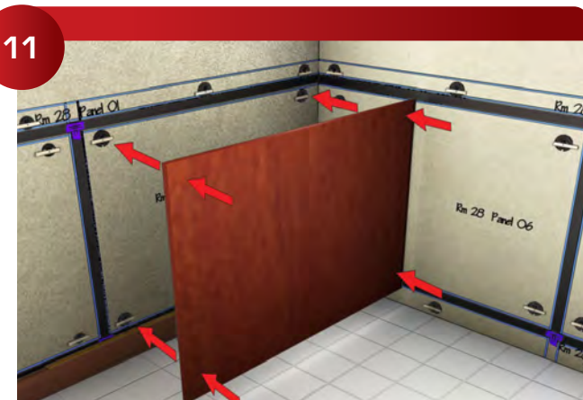
Carefully position your panel over your 211 Alignment Pins and push them firmly to leave a location mark for the 3/16" Mounting Screw.
