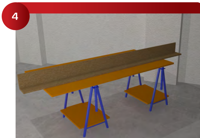
Preassemble the vertical furring corners (if any) and install them to use as a guide for the horizontal furring.
