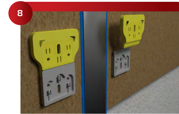
8 Place 410 NZ Alignment Clips on each individual panel's set of clips ( Tip: The 410 NZ Alignment Clips are reusable.).
