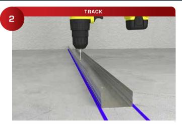
Butt all track joints. Securely anchor abutting pieces of track to a common structural element, do not splice or overlap because that bulges out the track.
