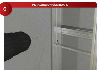
Use longest gypsum board length available, avoiding unnecessary joints. Do not use any gypsum wallboard that is distorted or wrapped. One side the wall with special specifications WD-1. Be sure to firmly screw all wallboard to the steel framing.
