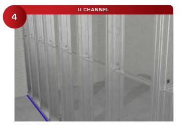
Use it least one row of cold-formed galvanized steel U Channel to hold the steel stud in place while installing the gypsum.
