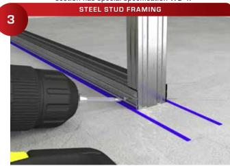
Use a #8 x 9/16 in. Waferhead low profile, self-drilling screws to attach steel framing. Do not use a standard panhead screw because they bulge out the gypsum wallboard.
