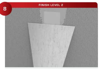
Locations to receive special specification WD-1 should have only a Level 2 finish. All joints and corners should have tape embedded in joint compound and wiped with a joint knife leaving a thin coating of joint compound over the joints and corners.
