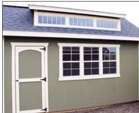
Shed dormer/ 3 windows
