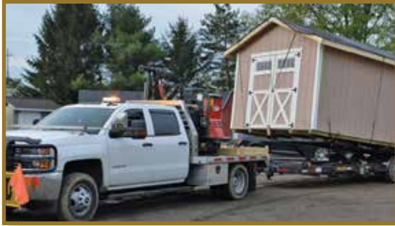
Pre-Built Barns delivered and set up on your prepared site
