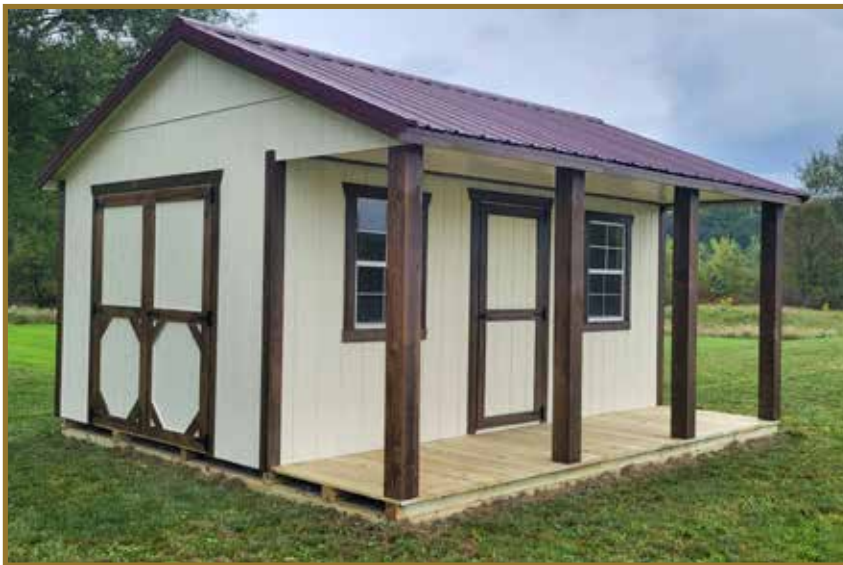
10' x 16' Cabin with these options: paint, extra window, metal roof & site prep.
