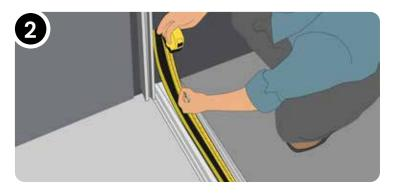
Use a pencil or marker pen to mark the desired length on the wrap-around seal, taking care to double-check all measurements.
