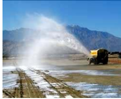
Construction Sites Fugitive Dust Control Erosion Control Road Stabilization
