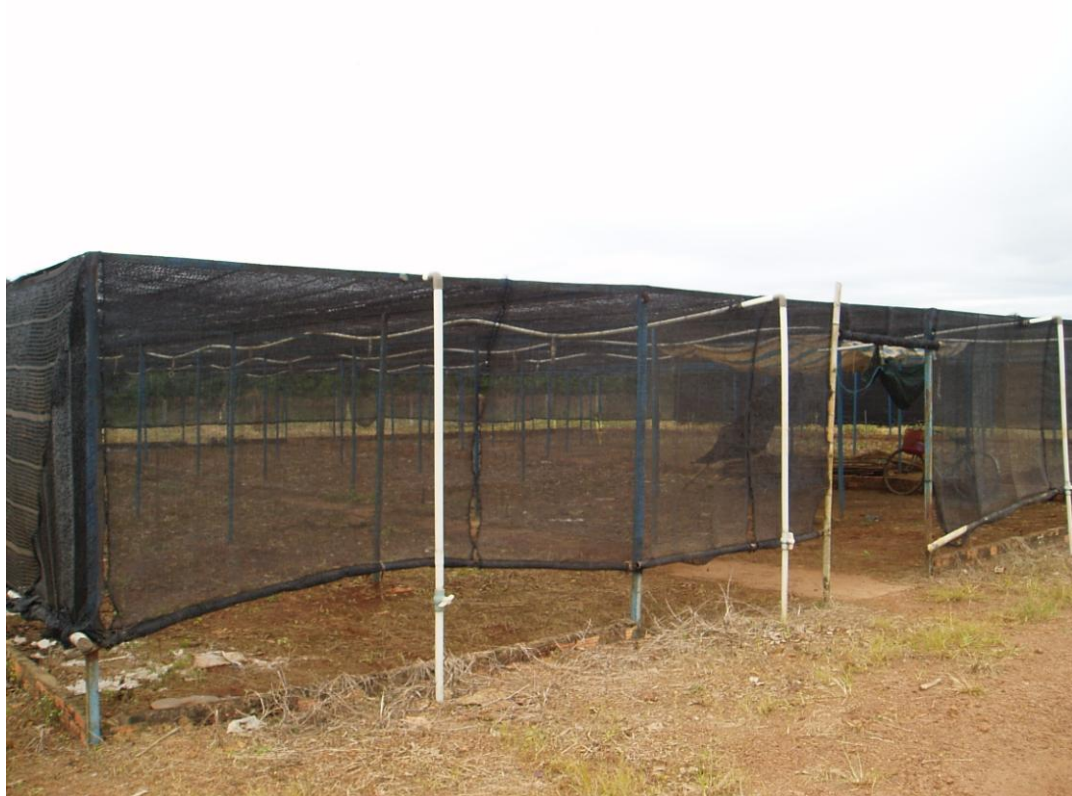
Photo 21: Using PVC pipes as scaffold and framework
