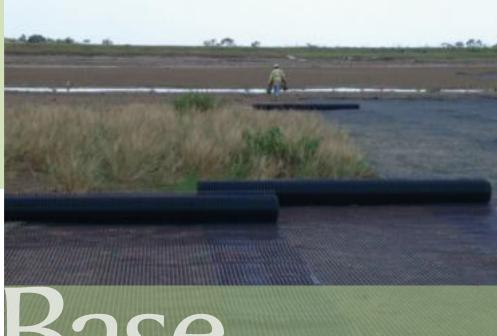
For 30 years biaxial geogrids have been utilized in pavement construction and soil stabilization projects throughout the U.S. and worldwide. StrataBase stabilizes aggregate/soil through confinement and introduces tensile elements, thereby increasing bearing capacity and load support capacity. StrataBase applications include:
