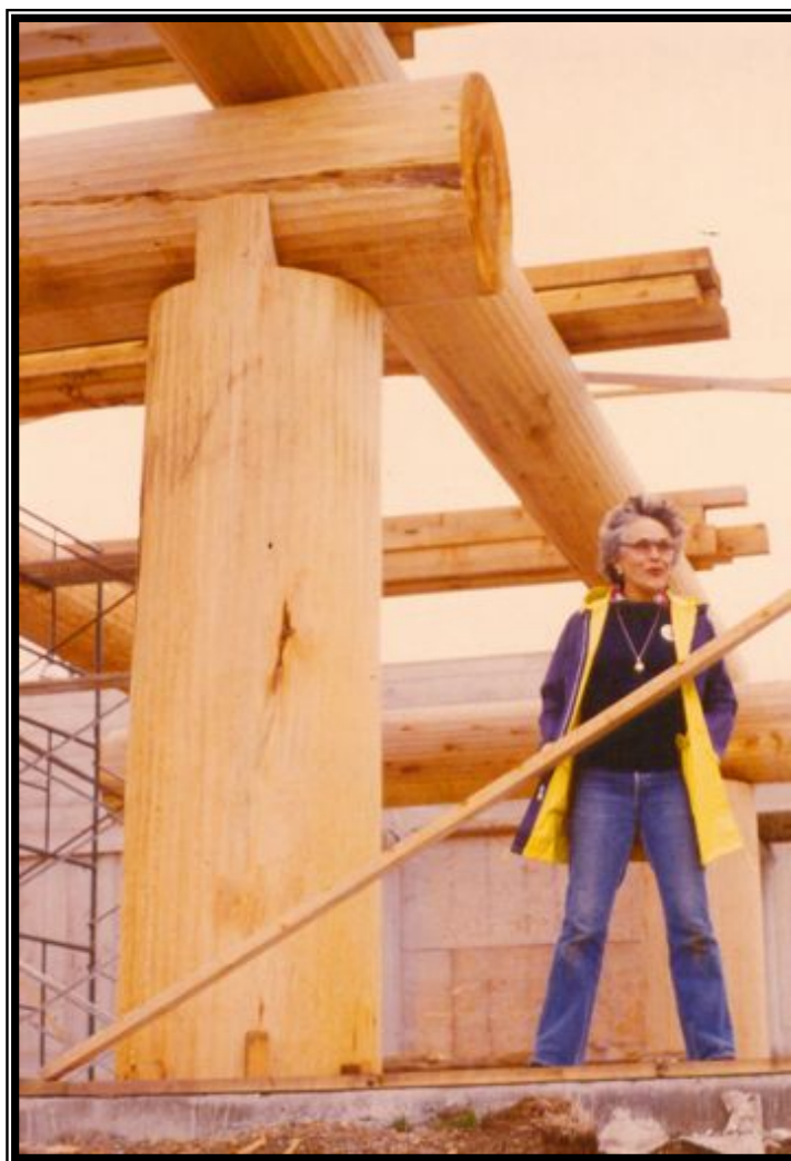
Gloria Webster on site building of U'mista Cultural Centre 1980
